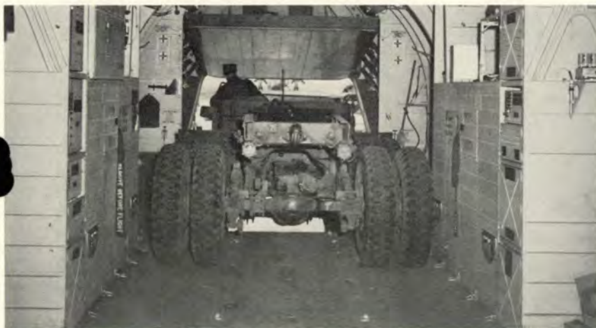
Wheeled vehicles and artillery pieces are loaded or unloaded without cargo handling equipment.
