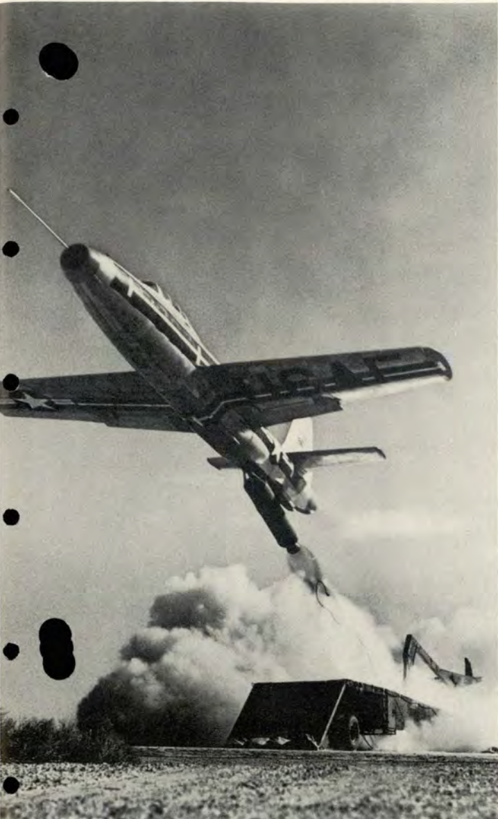
This jet, the first to take off from the highly mobile zero-length launcher, is propelled to flying speed by a droppable boost bottle.
